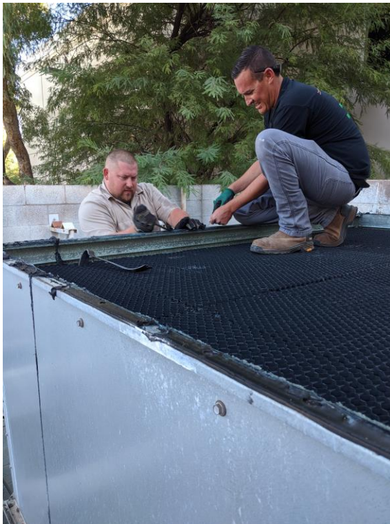
Old sealant was removed and replaced with fresh sealant before the new top was set in place.
