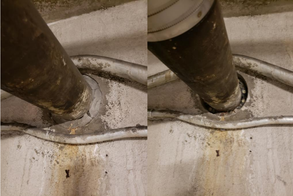
Picture of the 1 st pipe before, after old sealant removal, with 1 st coat of EP-990 Epoxy, then with 2K Epoxy top coat and then finally with Urethane Coating.
