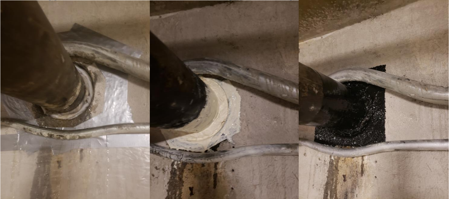
Picture of the 1 st pipe before, after old sealant removal, with 1 st coat of EP-990 Epoxy, then with 2K Epoxy top coat and then finally with Urethane Coating.
