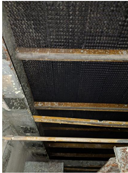
Media is in good shape only mild build up apparent.
