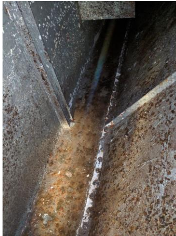
Media is in good shape only mild build up apparent.
