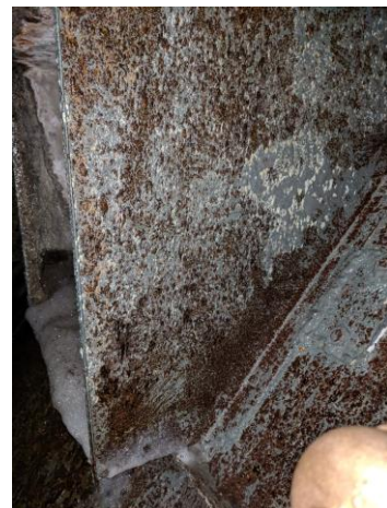
Several pictures of the heavy corrosion in the tower
