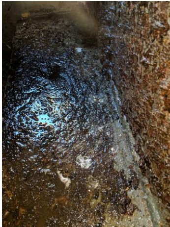
Media is in good shape only mild build up apparent.
