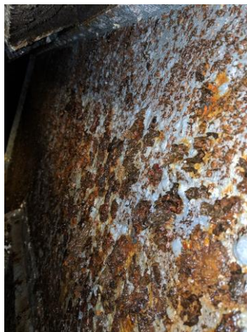
Several pictures of the heavy corrosion in the tower
