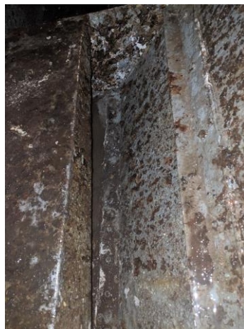
Several pictures of the heavy corrosion in the tower
